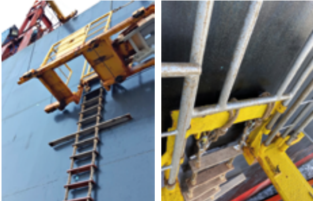
Dalawang (2) halimbawa ng non-compliant 'trapdoor' pilot boarding arrangements
