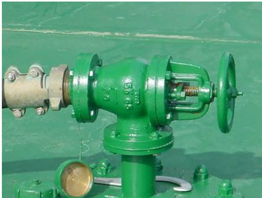
Figure 5 - Wilden pump discharge connection to slop tank
