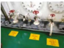
Quick closing valves in the engine room marked to help identify the valves during testing and operation.
